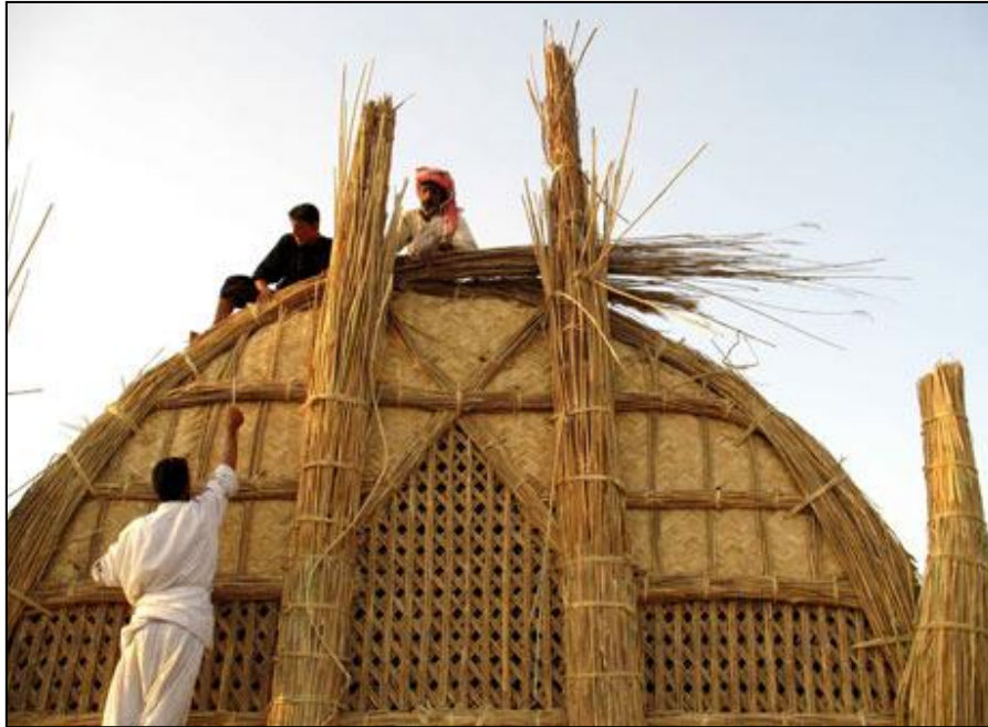
Construction of a 'mudhief' (reed house). Photograph: Mudhafar Salim/Nature Iraq
